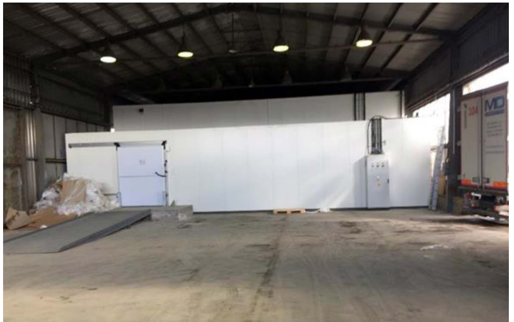
Fig.4: New cold storage build within an existing hall
