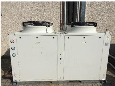
Fig. 1: Condensing unit
